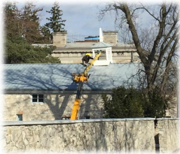
On the other hand, the workers from Harrison Bros. Construction waited until the weather warmed up. The snow needed to melt, and the roof had to be dry so that the cupola could be perched back on the roof. It had been removed in the fall while the Coach House asphalt roof was replaced with new prefinished steel roofing.
