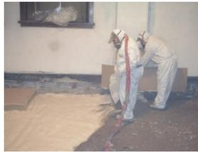
*After curing a two inch layer of spray foam was applied over the concrete.*
