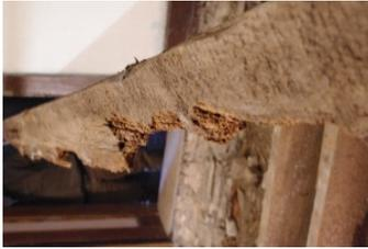
*In the Estate Office floor joists were rotting from the bottom due to moisture.*
