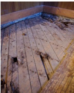
*To our surprise the billiard room tongue and groove floor was installed over a pine floor which was laid diagonally.*
