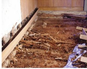
*Removal of floor boards revealed decayed conditions of the floor joists in the billiard room.*
