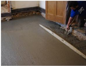
*After the dirt was levelled a four inch concrete base slab was poured.*
